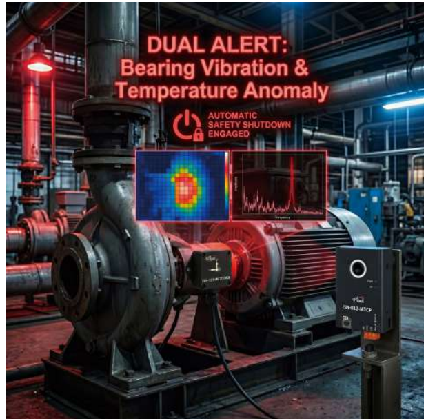
▲ Figure 4 | Predictive Maintenance Using Vibration and Thermal Imaging Combined vibration and thermal monitoring provides early equipment failure warnings.
