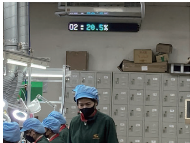
▲ The iKAN-124 displays on-site oxygen concentration.
