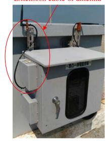
Fig. 2-2 Use extension cable of antenna
